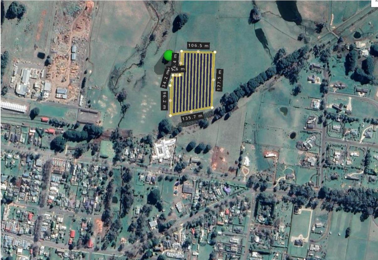
Figure 23: Power Station in Trentham
